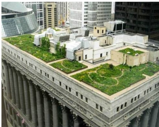
In 2001, a 20,300 square-foot green roof was installed atop Chicago's City Hall as part of the Urban Heat Island Initiative. When compared to an adjacent normal roof, City Hall's green roof was nearly 100 degrees cooler, and contributed to $5,000 in annual energy cost reduction. Photo: City of Chicago
