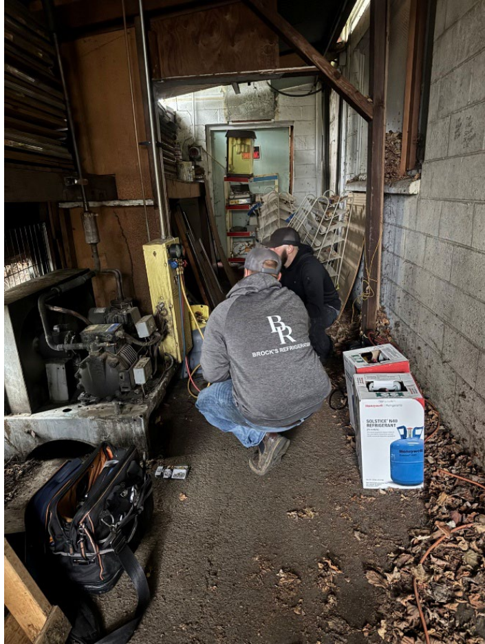
Replacing refrigerant on a walk-in cooler, Gilbert Street Market
