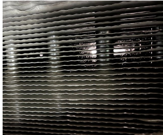
Before and after cleaning evaporator fins, Tom's Market
