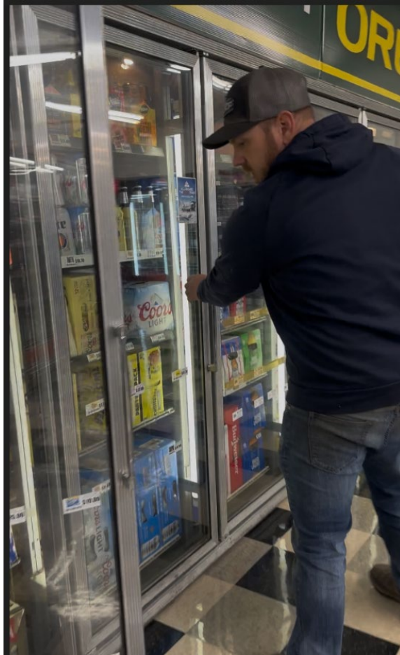
Replacing gaskets on fridges to improve door seals, Gilbert Street Market
