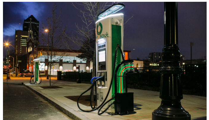
Charging stations for the first public DC fast-charging station for electric vehicles in Columbus, Ohio, lit up at night on January 14, 2019. The chargers are significantly faster and more convenient than conventional Level 1 or 2 chargers. The new charging station is a joint effort between Smart Columbus, the Columbus College of Art & Design (CCAD), the Columbus Foundation and Greenspot. CCAD students built a fiber-optic shroud to house the new chargers. Photo: Andrew Spear for NRDC
