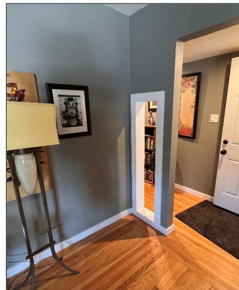
Image 5: Alpha and Pamela’s original natural gas wall heater was entirely removed.
