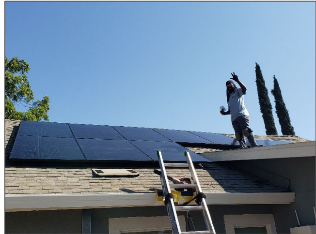
Image 2: Solar panels being installed on Marcisha’s new roof.
